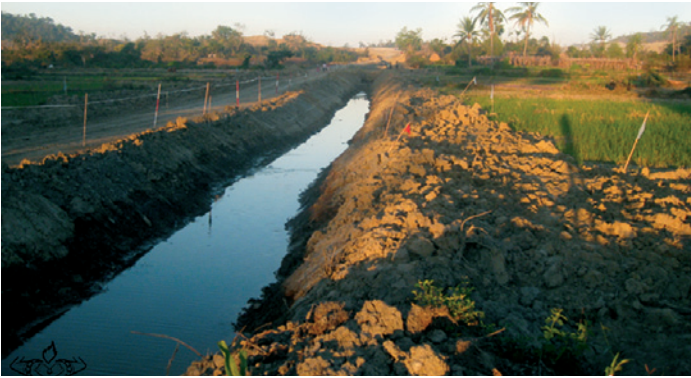
Shwe Gas Project cuts through local farms and prevents field drainage.
